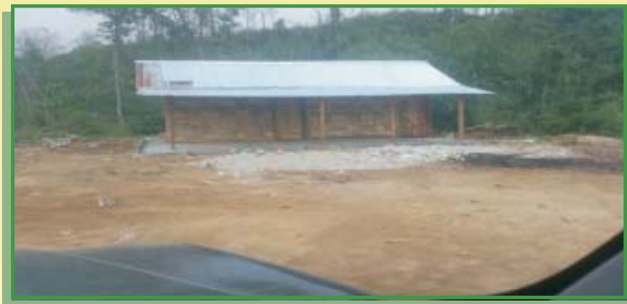
Temporary office-shed for supervising construction works at Jote
