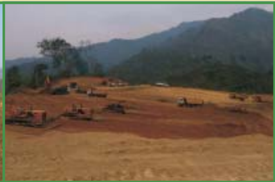
Site after levelling of land
