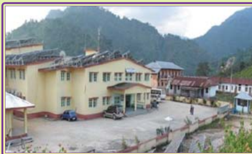
Solar panels on top of the building of NIT-Arunachal Pradesh
