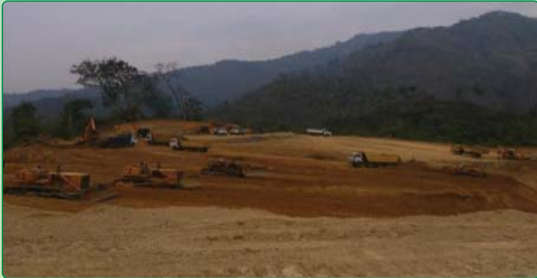
Site after levelling of land
