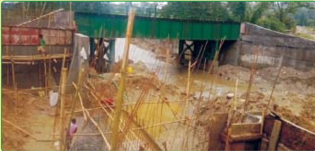
Steel Bridge at the entry of the permanent campus
