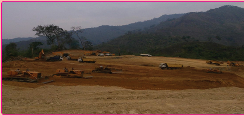
Site after levelling of land
