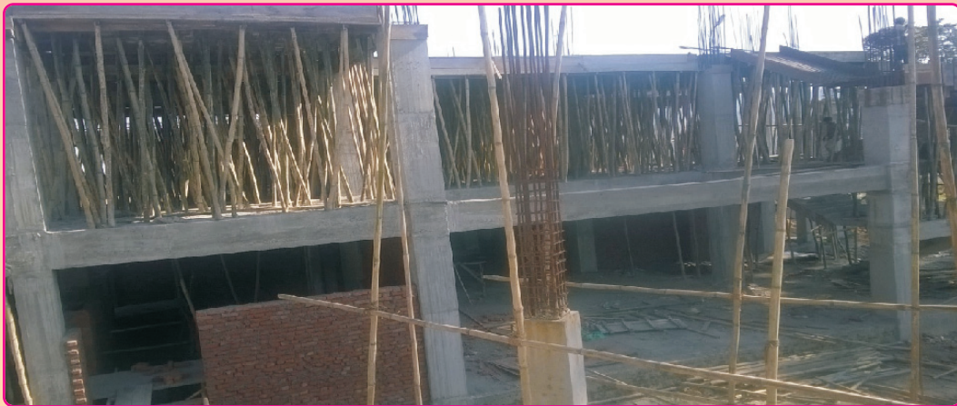
Academic Block: Civil Engineering Department.
