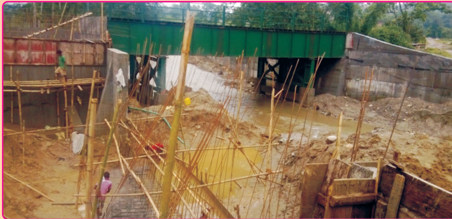
Steel Bridge at the entry of the permanent campus
