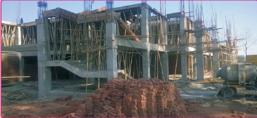
Academic Block: Mechanical Engineering Department.
