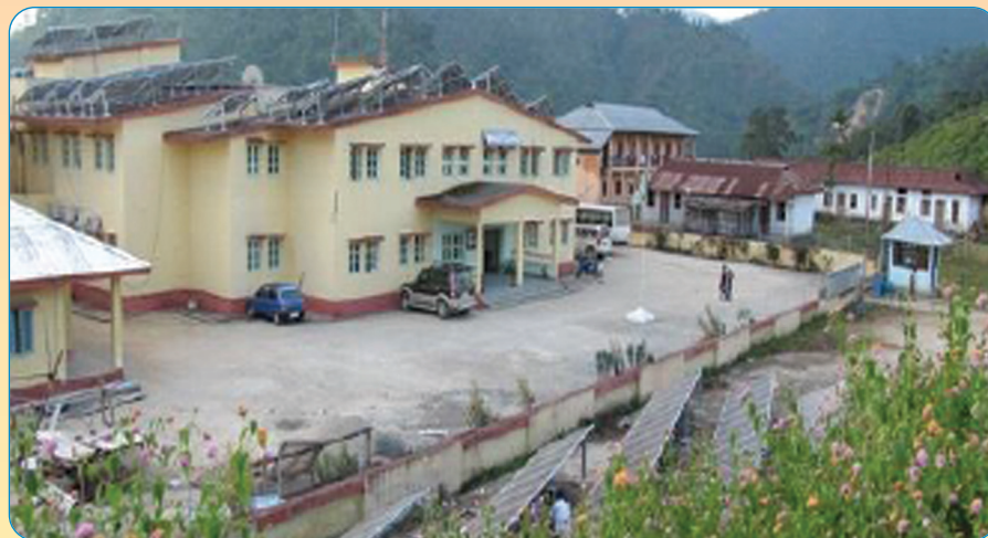
Solar panels on top of the building of NIT- Arunachal Pradesh
