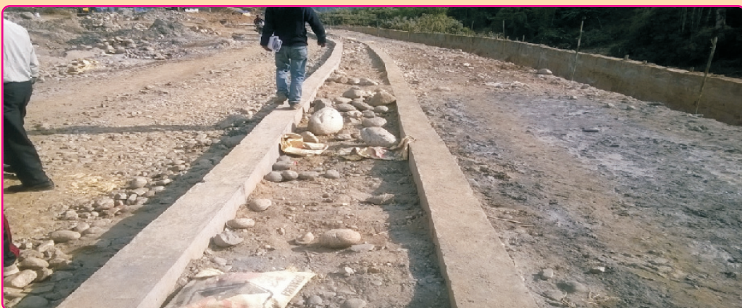
Campus Road and Drain
