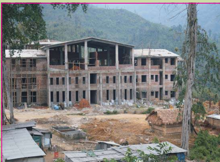
Civil Engineering Block
