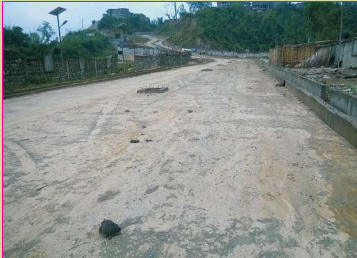
Feeder Road, main road and Internal Road
