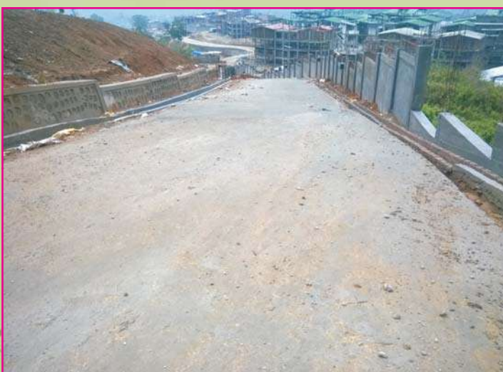
Approach Road to Water Treatment Plant
